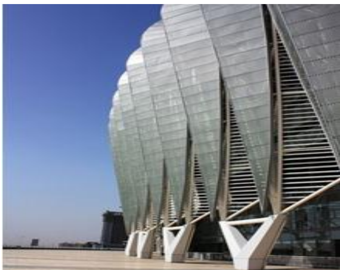
Fig 3: Shading System of Jinan Olympic Center Natatorium
